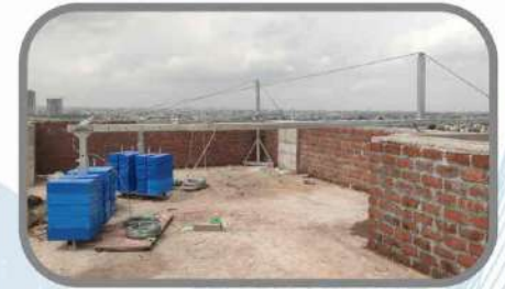
Terrace boom set with counter weight
